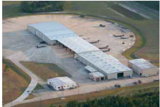
Fig. 1 The Gulf Coast facility
